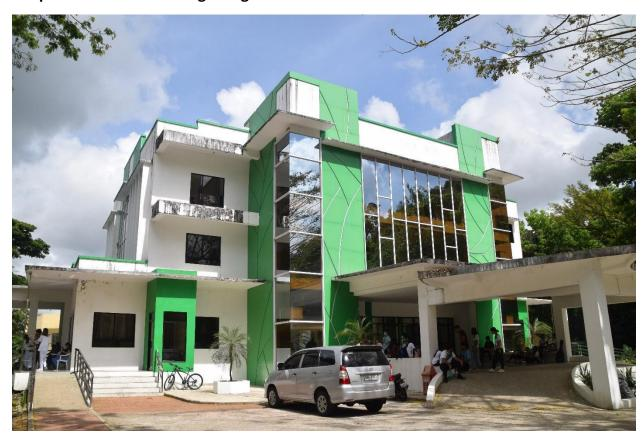
The Human Resources Management Center Building of the Aklan State University located at Banga, Aklan was designed to adapt Climate Change Mitigation (CCM) with large glass windows to reduced extensive lighting, and allows fresh air ventilation.
